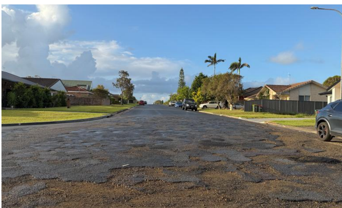
Figure 8: Sight Line Looking North
